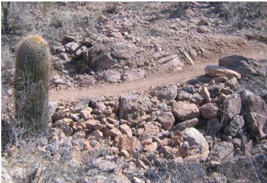
A crib wall raises the bottom of this drainage, eliminating a fall-line drop into the wash. Rocks piled against the base of the crib wall prevent undercutting as the water flows over it.
